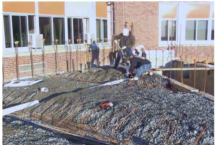
Figure 1: Areas Isolated by Thickened Slabs
